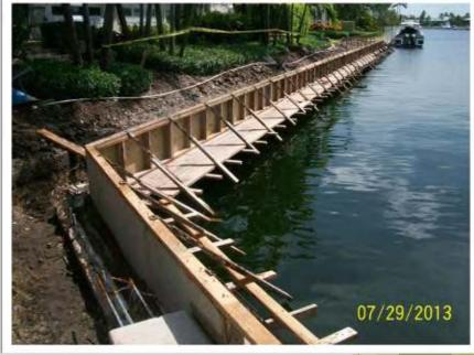
These photos show a cap replacement in progress. The seawall panels and pilings were in good condition, but the cap was badly spalled and needed to be replaced. The outer cap form boards are in place and you can see the tops of the seawall panels and "T-pilings". Notice how there is rebar protruding from the top of the seawall panels and pilings. When the cap is poured it will connect all of the seawall components together into a solid homogenous structure.
