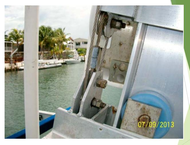
Cables are only as strong as the connections that hold them together. Look at the condition of the compression or bolted cable clamps for excessive corrosion or signs of cable damage at the connector. A lift cable may look perfect until you see how it is connected. Watch for amateur clamps, I have seen automotive bull-dog clamps used!
