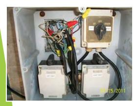
Be sure to check the condition of electrical cables and wires. Report any spliced or wires in poor condition.
