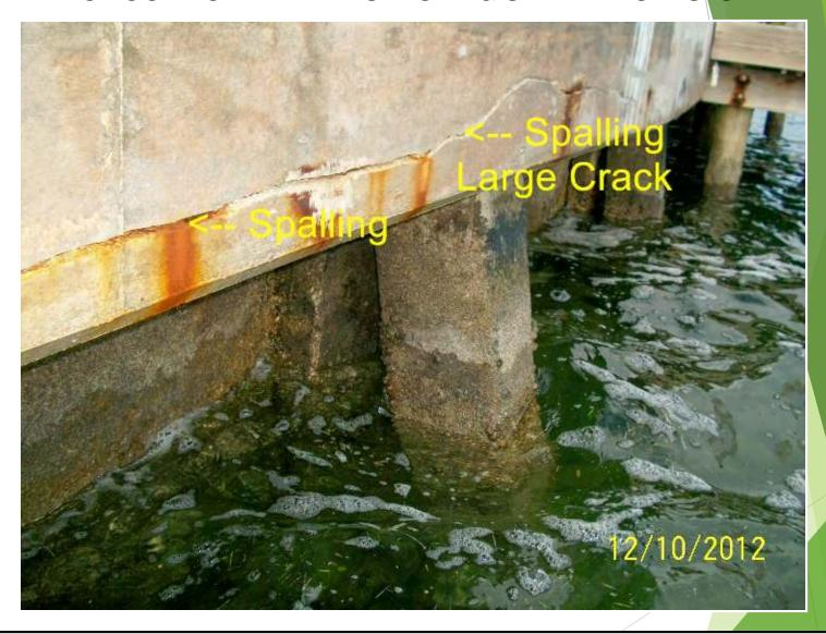
This cap shows significant spall cracking. Notice that the cracks have been "patched" by filling the cracks with grout. This is not a proper repair, repairs will be needed.
