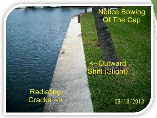
Always remember that form carpenters like to build things in straight lines! It is difficult to bend forms to make curves. If you look along what should logically be a straight seawall and it is curved, there is a chance of outward movement. Outward movement could indicate failed tie back anchors.
