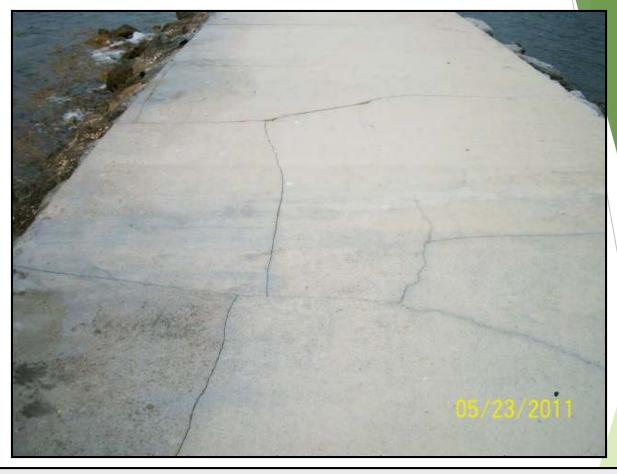
Concrete docks are susceptible to cracking due to settlement or shrinkage just like any other concrete slab. Be sure to use good judgment to determine the cause of cracking. In the case of this photo, the cracking is normal shrinkage cracking since no control cuts were made to control the shrinkage. In this case the cracking is a minor cosmetic concern with very limited chance of being an ongoing concern.
