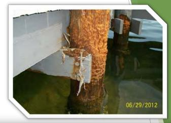
Pilings are "legs of the table" that hold the entire wood dock structure up. Pilings can be damaged from vessel impacts, rot/fungus or deterioration below the water line. If possible try to look down into the water to check for "thinning" of the pilings.
