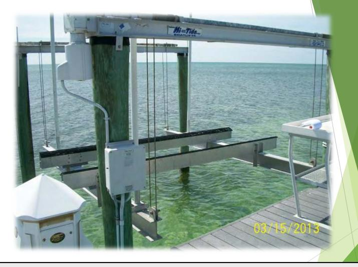
Overhead beam lifts have lift bunks that are suspended by cables at all four corners which are connected to a rotating winder bar. Overhead beam lifts are installed across pilings on each side. Maximum capacities for these lifts typically range between 4,000 lbs and 16,000 lbs.
