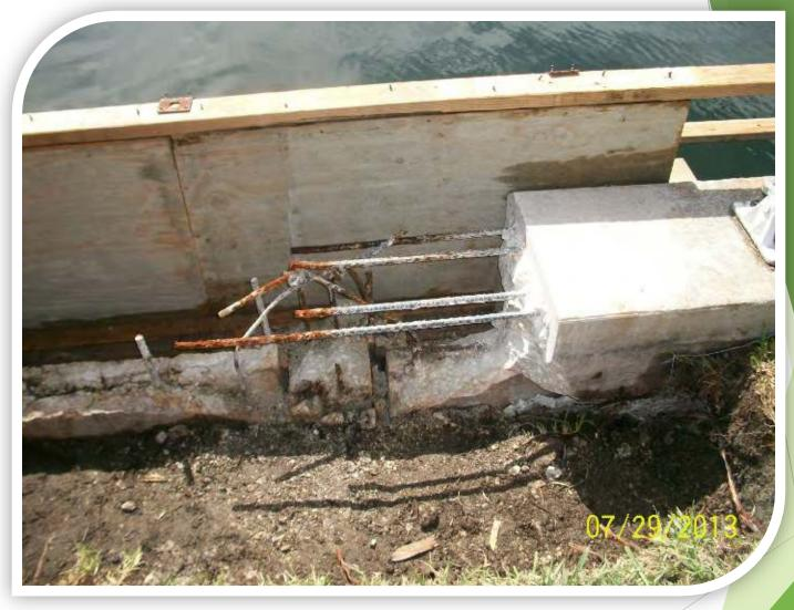
A seawall cap is basically a tie beam as you would see in any masonry CMU constructed home. The seawall cap "ties" the seawall panels and pilings together and provides a rigid diaphragm to help keep the seawall straight.
