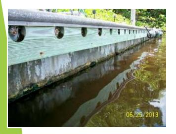
Inspect the condition of the banding board bolts, nuts & washers as well as the condition of the wood bands.
