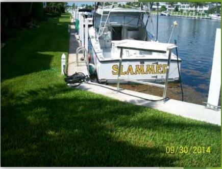
These photos show the finished repair from the previous slides. Notice the level of the landside fill and grass. It is important that the grade be high enough to not allow too much water to get trapped landside of the seawall. Ideally, water should flow over the top of the seawall cap during heavy rains. Some seawalls will have a French drain to help with drainage. If you notice excessive difference between the land elevation and the top of the cap, expect to find erosion problems.
