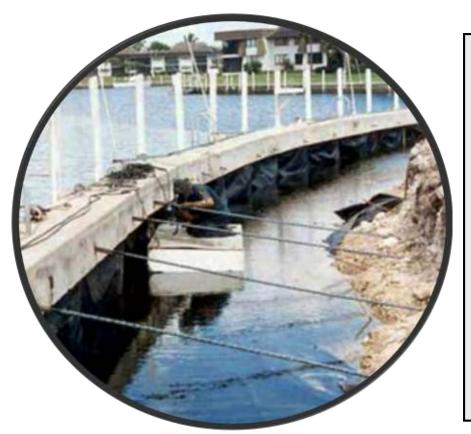
Tie back or "deadman" anchors are steel rods that connect either through the seawall cap, seawall pilings, or in rare occasions, through the seawall panels and anchor into the ground. These tie back anchors help to prevent outward movement caused by the pressures of the landside fill against them. Tie backs are critical to the stability of seawall structures. However, some seawalls do not have tie backs, usually shorter or inside curved seawalls do not need them.
