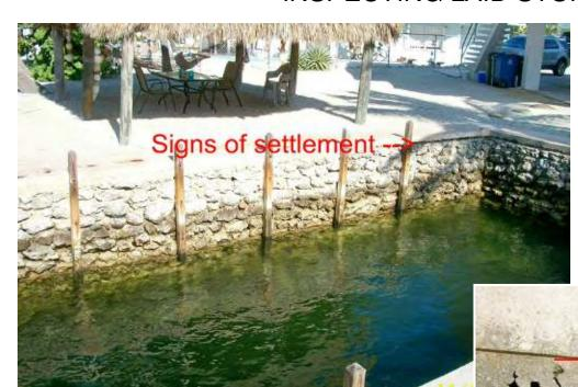
Look at the seawall from a distance if possible to see any irregularities. In this instance you can see the line below the dock slab dropping off toward the corner.
