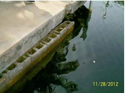
When inspecting masonry CMU seawalls look at the mortar joints and connection to the dock slab or cap for signs of settlement.
