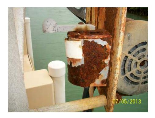
Any rusted or broken switches or exposed wiring needs to be reported. Just use the same FABI protocols you would use for inspecting the electrical within the home.
