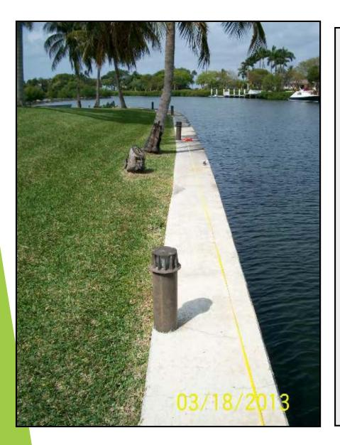
As mentioned in the previous slide, this seawall was bowing due to excessive land fill which was put in to elevate the home for a better view. The soils created so much pressure that it shifted the entire seawall structure, AND even shifted the tie back anchors.
