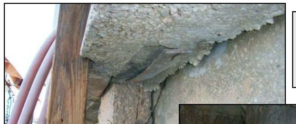
In these photos the seawall structure is still stable, but repairs will need to be done at some point in the future.
