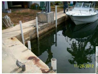
Masonry CMU seawalls are basically a block wall on either a footer or natural rock.
