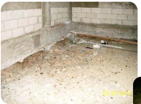
After realizing that soils pressure was causing the seawall panels to shift I looked in the crawlspace of this home to see if there were any indications of settlement.
