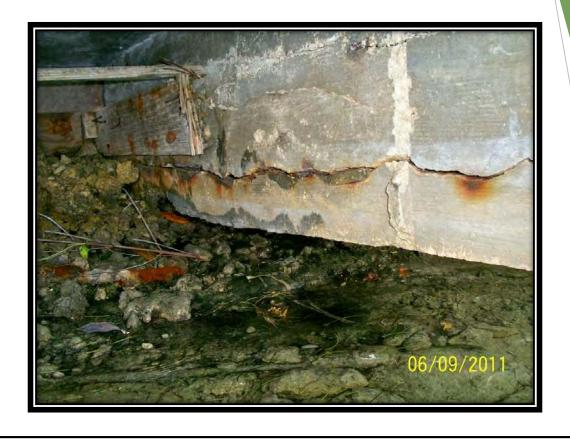
A natural repose seawall is basically any shoreline that has not been improved that supports or is below another dock structure. This photo shows a concrete dock support beam that appears to be resting upon the natural ground. Our concern for this discussion is not the beam, but the condition of the natural soils. In many cases the "natural repose" is actually just a beach as you would see with a finger pier that extends out into the ocean or a lake.
