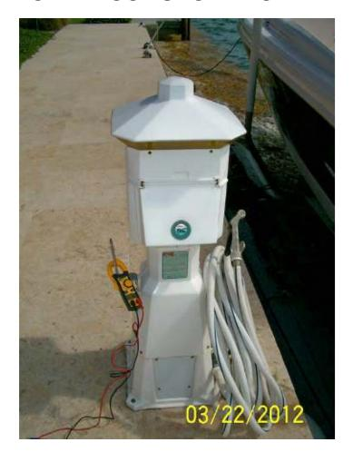
Inspect a shore power pylon just like you would any panel or sub-panel. Expect to find a 20-amp (120-volt) GFCI outlet, a 30-amp (120-volt) marine outlet, most times a 50-amp (240-volt) marine outlet, and occasionally a 100-amp (240-volt) or larger marine outlet. All of these circuits should have their own breakers at the pylon.
