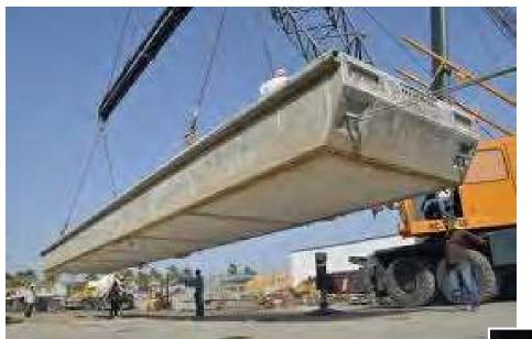
Although it seems illogical that concrete can float, it does. Floating concrete docks are made from huge Styrofoam blocks that are encased in concrete on all sides except the bottom. These floating docks can be massive structures.
