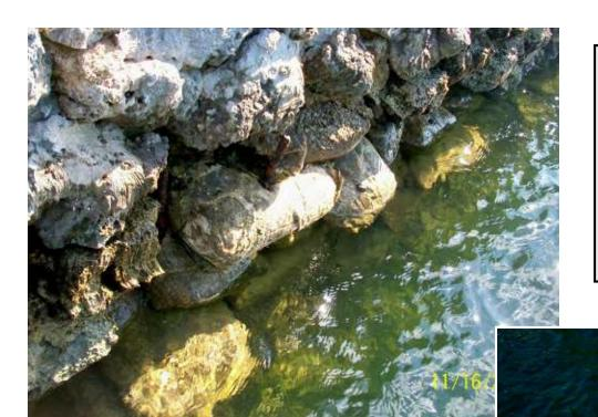
Past repairs are clear indicator of potential problems. This wall was patched with concrete sand bags because the soils behind washed out taking the seawall with it. Be sure to list previous repairs on your report.
