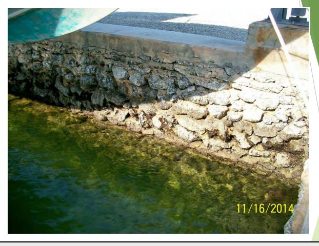
Laid stone seawalls require a lot more attention than masonry CMU walls due to the non-linear structure. This section of seawall is in pretty good condition with no signs of settlement or cracking. Look very closely for voids, past repairs and especially settlement. Settlement indicates failure or erosion of the foundation.
