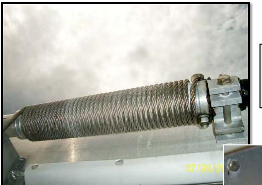
Always check to make sure that the lift cables are wound-on to the winder bar or spool as evenly as possible.
