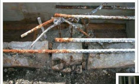
Looking closely you will be able to see the top of the "T" piling and the rebar protruding from the top of the piling. After all of the steel is installed it will tie all of the seawall components together.
