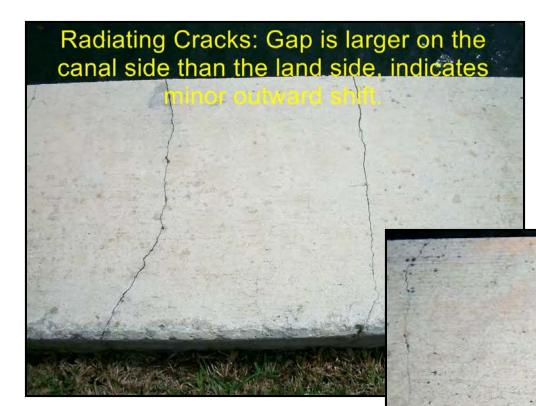
When a cap has cracks that are larger toward the water and tight at the land side it indicates outward movement of the cap and seawall.
