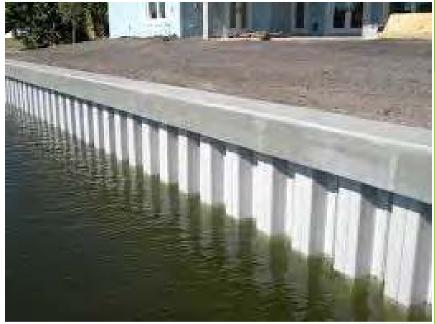
Although not as common as steel sheet pilings, plastic sheet pilings do make a very clean looking, low maintenance seawall. The reason they are not as common in South Florida is because of the limestone substrates in our area. Plastic sheet panels may be more common in areas where the ground is not so hard.
