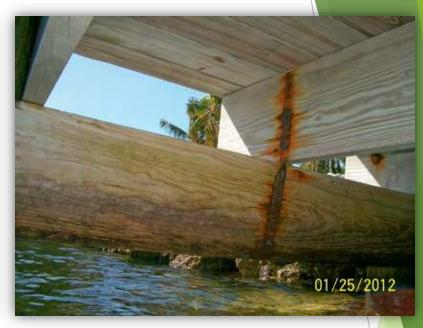
Anchors, bolts and straps make up the ties that hold the dock structure together.
