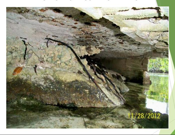
Looking below the dock it is apparent that there is no longer any support for the dock structure. This is a MAJOR concern because not only does the seawall need to be replaced, but the dock structure needs to be stabilized as well.
