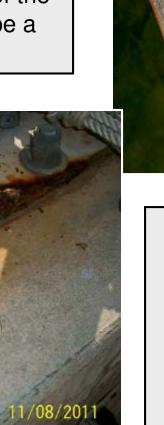
However, this rust has migrated into the bolt hole location and you are seeing the rolled steel layers indicating serious rust. This base MAY be repairable, but the entire davit base stanchion will likely need to be replaced. If allowed to worsen, this base plate could fail.
