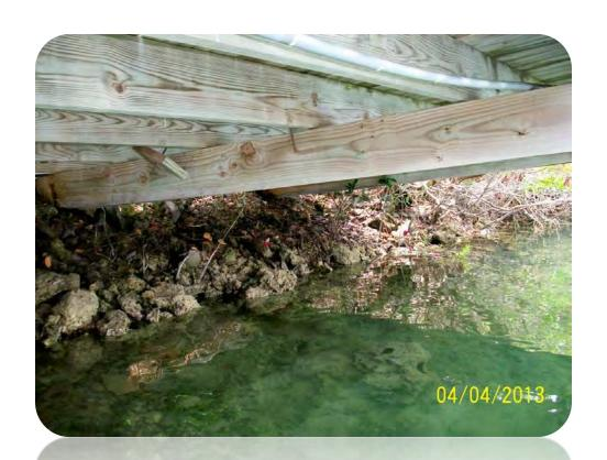
As stated in the previous slide, a "natural repose seawall" is not actually a seawall, but land that is unimproved which, in some cases, MAY support the structure of a dock.
