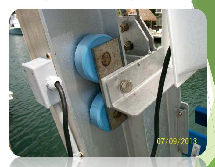
Inspect side elevator lift rollers for condition and lubrication. Watch the rollers while operating the lift to make sure that they are turning. Any frozen rollers should be reported. Always recommend lubrication if questionable.
