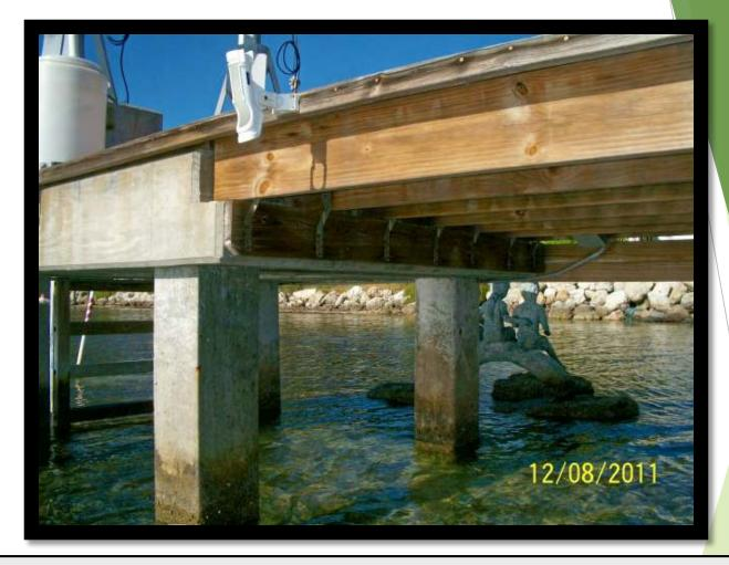
Just as you would inspect any deck on a home, the connection of the wood dock to the landside structure or concrete dock is critical. The dock/joist structure MUST be supported with sufficient lag or anchor bolts, or as in the case of this photo, a ledger as well as bolts. Docks can collapse just like a residential deck can. Be diligent on checking for proper structural support and bolting below.
