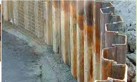
Sheet pilings are interlocking corrugated steel or plastic sheets that are driven into the canal bottom vertically creating a seawall face. Usually the sheet piles are capped with a traditional seawall cap to keep the wall straight and even.
