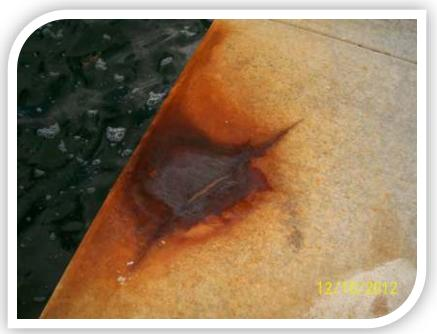
In many cases rust bleeders are just moisture that wicks into the concrete due to hydrostatic pressure coming into contact with the rebar causing rust stains. This is VERY common when the dock is a slab-on-grade and there is a step-down from the landside with elevated lawn areas etc.. This is considered a cosmetic concern that should be monitored.
